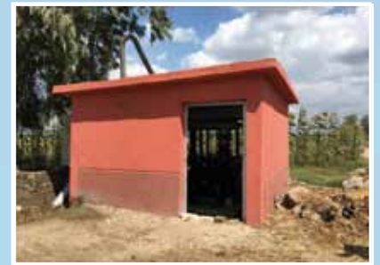
Pump room in Egypt
